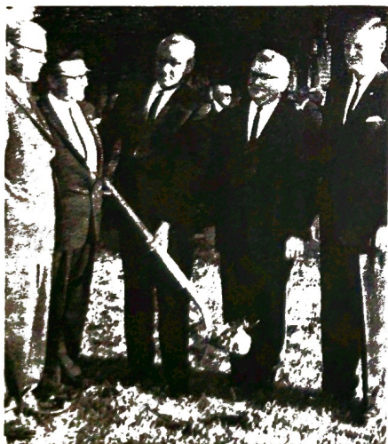
Taking part in ground-breaking ceremonies at Scottville are, left to right: Robert Nelson, contractor; Rev. Heath T. Goodwin, superintendent, Grand Traverse District; Max Keifer, chairman, Building Committee; Rev. Kenneth L. Snow, pastor; and Robert Miller, mayor of the city of Scottville.
